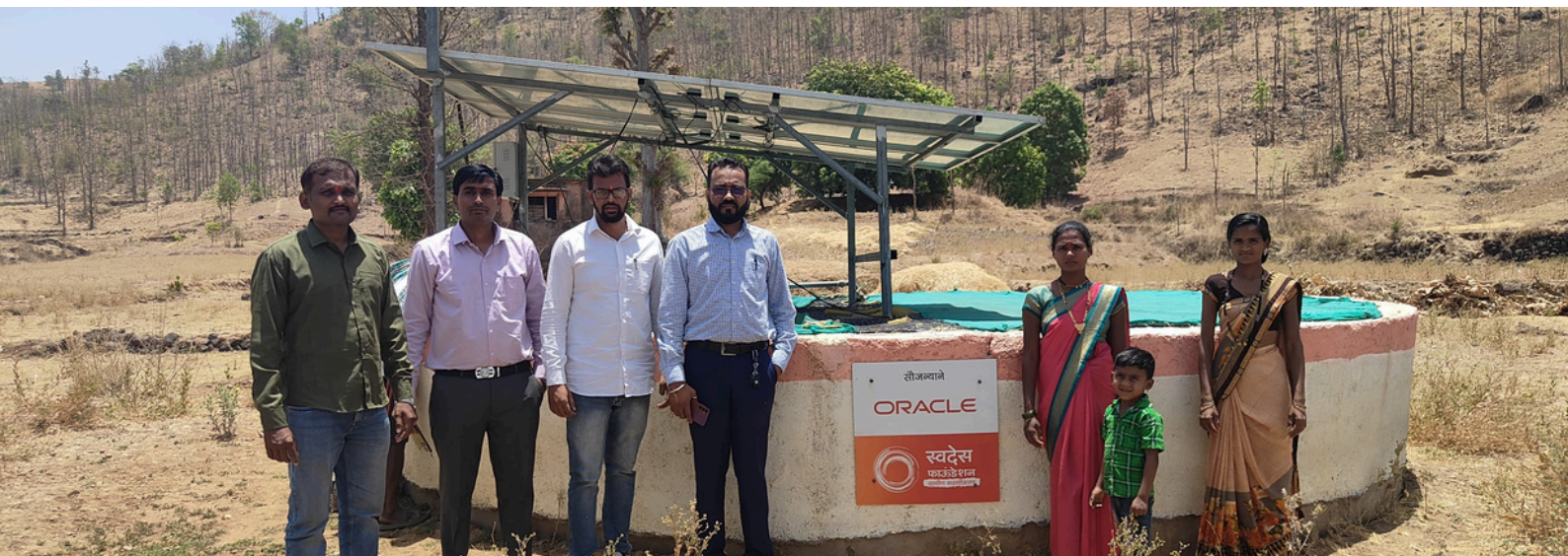
DRINKING WATER WELL RENOVATED AT HATHRUNDI VILLAGE
