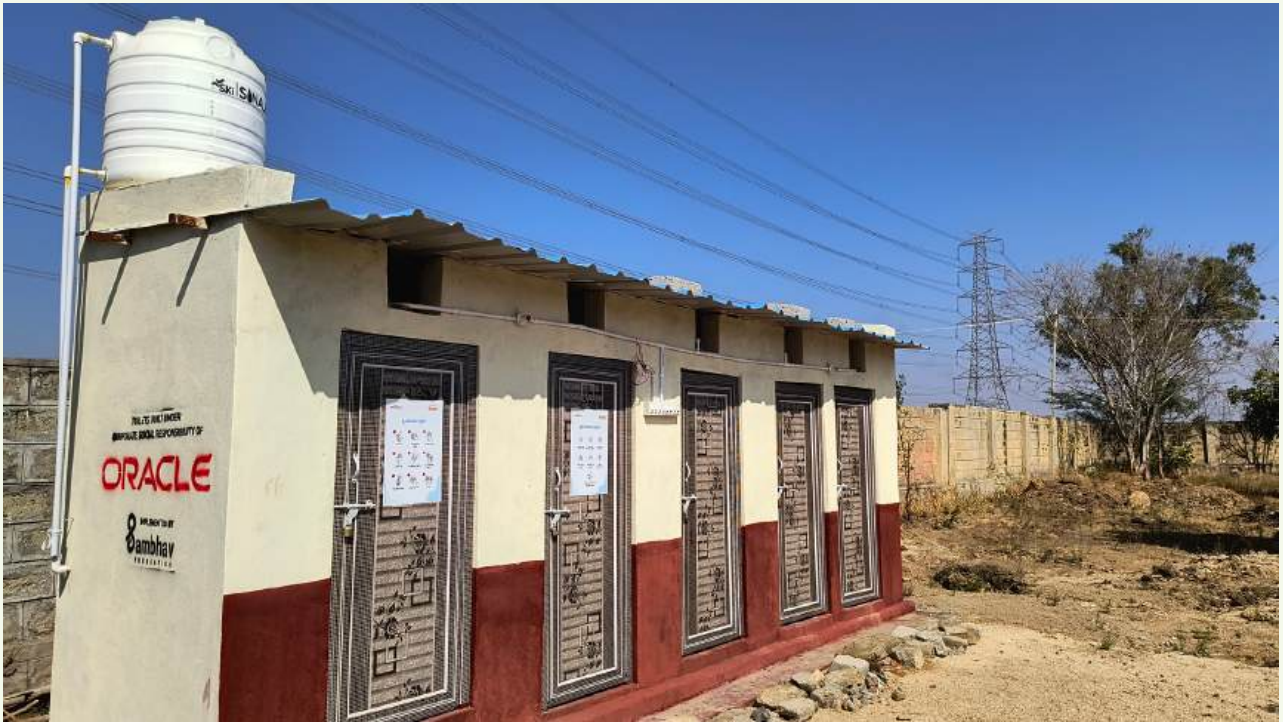
Newly constructed sanitation facilities constructed through the Sambhav Foundation project
